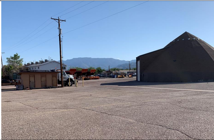
Salt Storage Building
